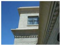
Custom produced Eave Moulding manufactured in Fabric Reinforced Concrete. Supplied and installed by Old World Concretes (Pty) Ltd
