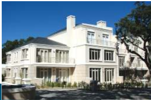
Custom produced FRC Mouldings supplied and installed by Old World Concretes: 1st Floor, 2nd Floor and Eave.
