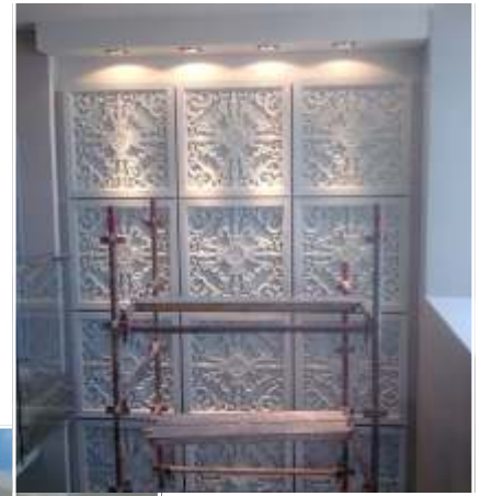
Decorative Panels to architects design supplied and installed by Old World Concretes at One & Only Hotel
