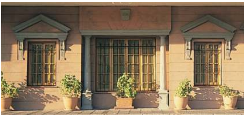
Apex Pediments with Scroll Corbels, Type 86 Columns on Beaded Pedestals with Paris Lintel over.
