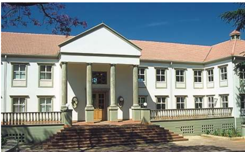
By Old World Concretes. In-situ cast columns, Woodlands Lintels, Number 13 Balusters with plinth and coping.
