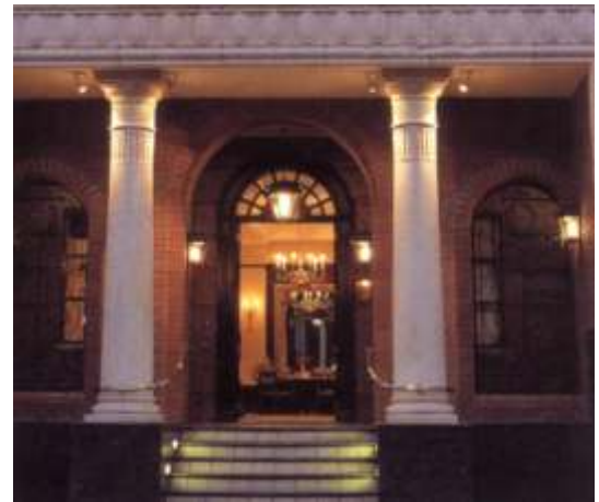
In-Situ cast columns supplied and installed by Old World Concretes (Pty) Ltd.
