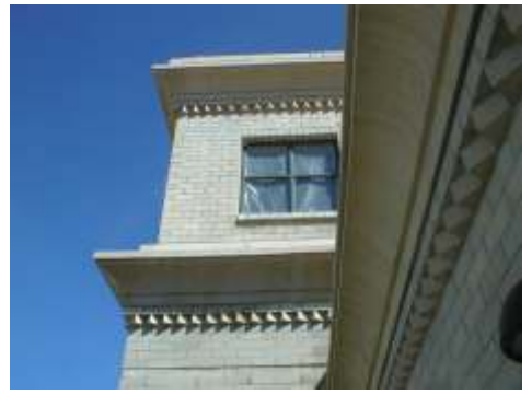
EAVE MOULDING: In Fibre Reinforced Concrete. Supplied and installed by Old World Concretes.
