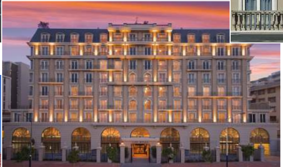
WINDOW SURROUNDS: In Fibre Reinforced Concrete. Supplied and installed by Old World Concretes.
