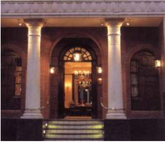
In-Situ cast columns supplied and installed by Old World Concretes (Pty) Ltd.
