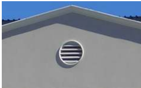
LOUVRE GRILLE 750mm 750mm diam x 260mm deep (in two pieces)
