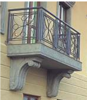
WATERHOUSE SCROLL TRUSS 920mm high x 820mm deep x 450mm wide.
